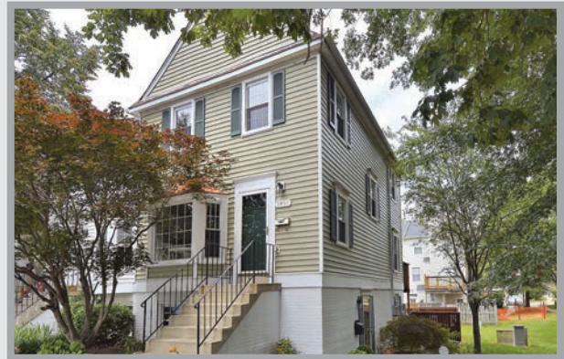
PIGGY-BACK TOWNHOME: A townhome structure that is divided both horizontally and vertically, consisting of a single level, lower level unit, with a 2-story upper level unit.
