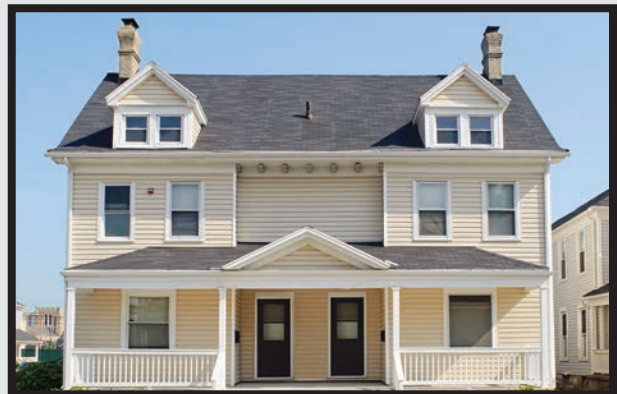
DUPLEX: A type of semi-detached home consisting of two separate living spaces attached by a common interior wall.
