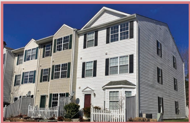
BACK-TO-BACK TOWNHOME: A type of townhome where the backs of two different units share a common rear wall, so that neither unit has a backyard or rear facing windows.
